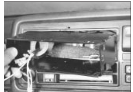
31.6 Radio/cassette container removal
