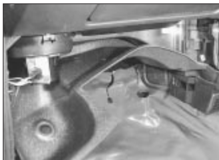
8.6b . . . and insulation sheet
